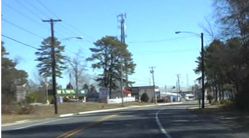
Communication tower at Giffordtown Road, Little Egg Harbor Township, viewed from US Route 9 eastbound
